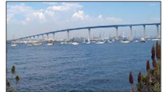
Steel Box Girder
